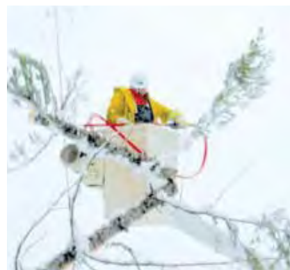
Power line technician during a Campbell River snowstorm.
